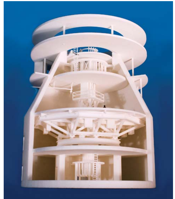
An SLS model showing the cutaway view of the internal structure found inside the ATST building. The telescope assembly will be mounted on the top platform. A rotating lab is located inside the pier and can be seen directly underneath the telescope mount.
